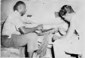
As part of the expansion of the new telephone facilities, D. Mitchell and G. Arends splice cable in the refinery.
